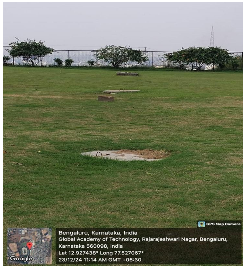
Figure 7-2: Rain Water Harvesting Pits
